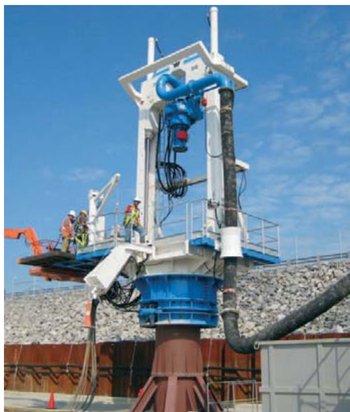
The Wirth drill being installed atop casing bolted to the work platform at surveyed locations
