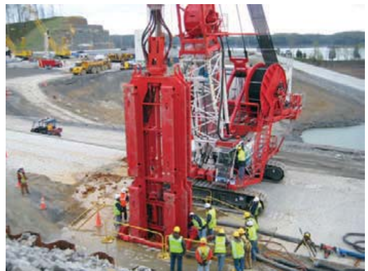
The hydromill is inserted into a steel guide frame locked into guide walls on the work platform, allowing the mill to begin excavation at the right location in a vertical position
